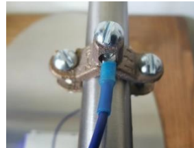
proper pipe clamp attachment
