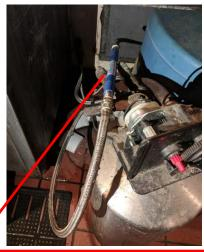
NaturalSof Pro installed and other filters/treatment removed NaturalSof Pro installed and softener disconnected
